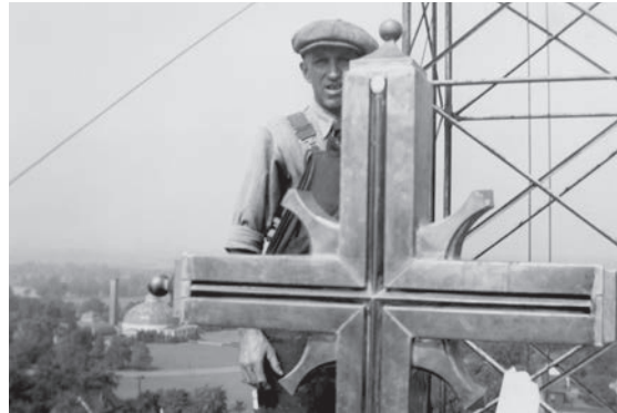
Local tradesmen were involved in every aspect of construction.
